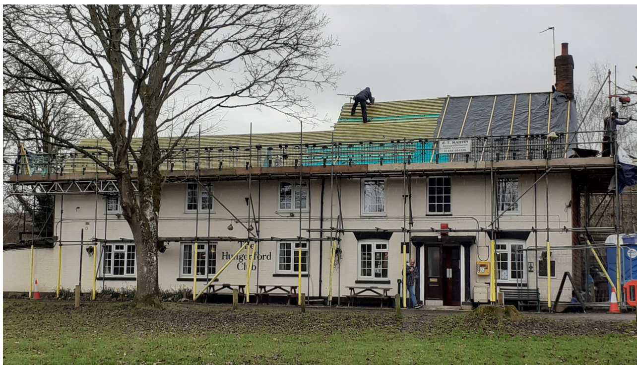
Work in progress to renew the club roof - March 2023
